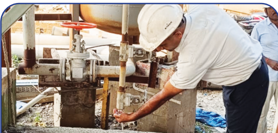
KGEPL Hazira Bio-Ethanol Plant Boiler Flushing Starts – 26 th December, 2025
